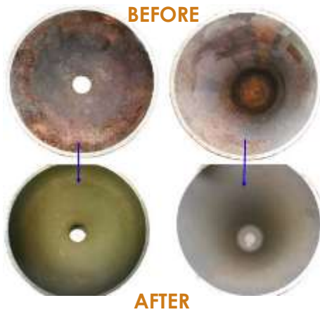
Cylinders before and after cleaning
